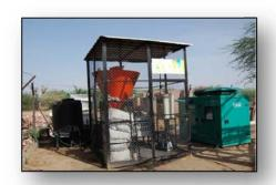
The start-up proposed a technology that converts biomass into a gaseous fuel used to power an internal combustion engine that turns a small electrical generator. The start-up believed that this system could replace the diesel powered generators at an overall lower cost per kW/h.
